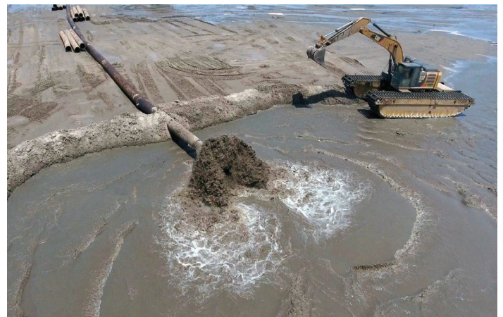
Dredge materials have been used to help rebuild coastal Louisiana. P.J. Hahn, Pelican Coast Consulting and the Big River Coalition.
